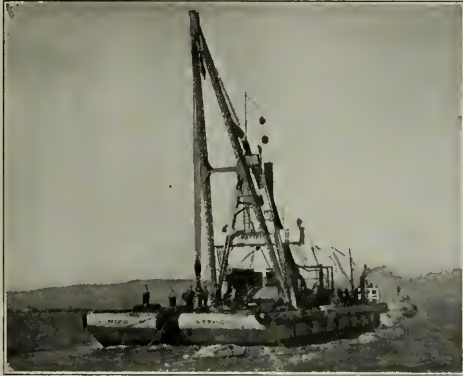
Pacific Telephone and Telegraph Co. Cable Barge. (P. T. & T. Photo.)
